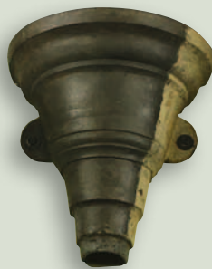
An interesting example, c.1795–1810, with a 'D'-section downpipe, possibly originally made of lead. The elegant design closely follows the detailing of late 18th century examples, but on a much smaller scale.
