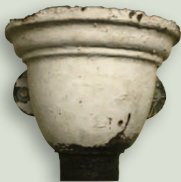
An early cast-iron version, following the traditional lead form but on a smaller scale, c.1825–35. The fixing lugs forming part of the casting.
