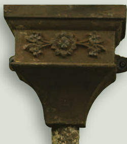
A good example of restrained naturalistic ornament on a cast-iron rainwater head of the early 19th century.
