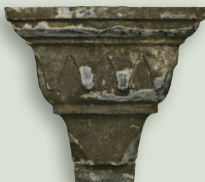
A cast-iron design of the c.1820–45 period. This example was fixed directly through the back-plate of the rainwater head.
