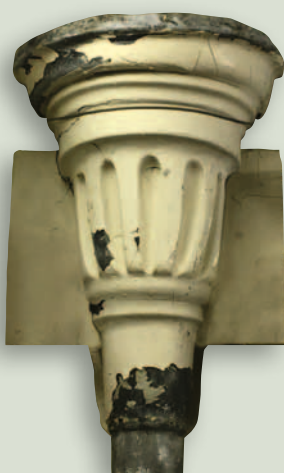
Fine late 18th century widely used rainwater head pattern. Typical of designs that have been dressed over a wooden former-block.
