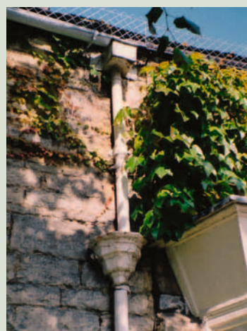
A combination of lead and cast-iron rainwater goods, c.1820–35. Note the simple lead box design (top) with rolled moulding to the upper edge. The cast-iron rainwater head (below) is a faceted design widely used from the early 19th century until the early 20th century.
