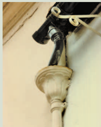
A fine example of an ornamental semi-circular tapering cast-iron rainwater head, c.1820–50.
