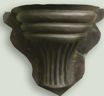
Sheet copper rainwater head, late 18th/early 19th century. This design was almost certainly worked around a wooden former-block, as with lead varieties.
