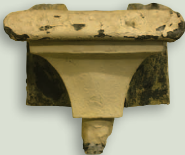
Simple lead rainwater head, c.1810–28, from Woodhill Manor, Shamley Green, Surrey.
