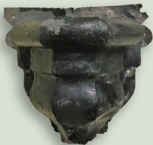
Zinc rainwater head, c.1820s–30s. This is constructed of zinc sheet sections soldered together.
