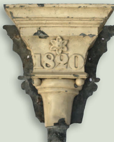
Lead rainwater head. Note cast lead floret and spheres, the numerals were cut from lead sheet.
