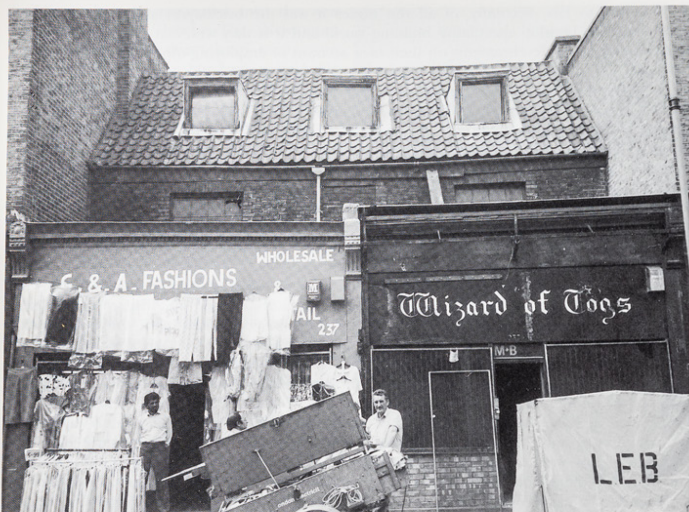
Fig. 6. No. 237 Hoxton Street, early eighteenth century, prior to restoration
