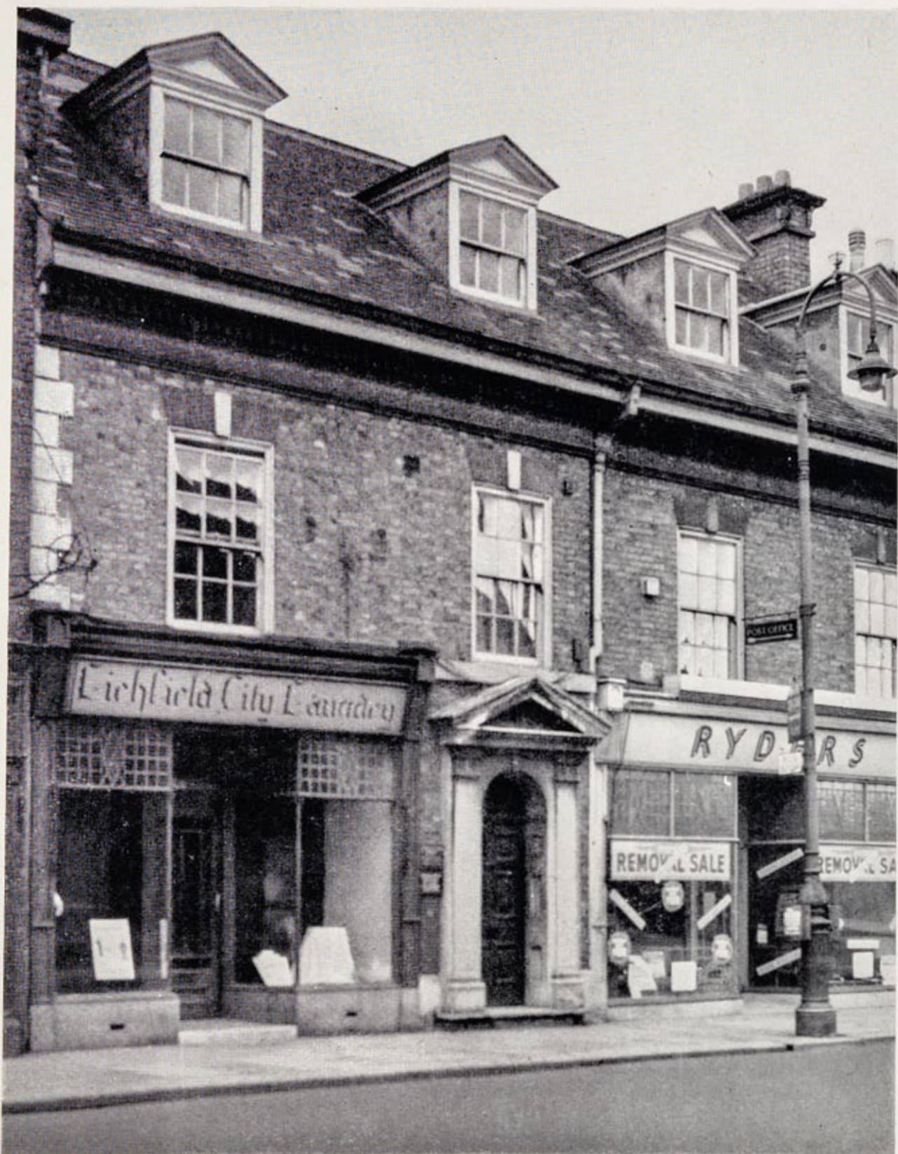
A good Georgian building poorly adapted to commercial use. There is little to be said for the lettering of either of the fascias.
