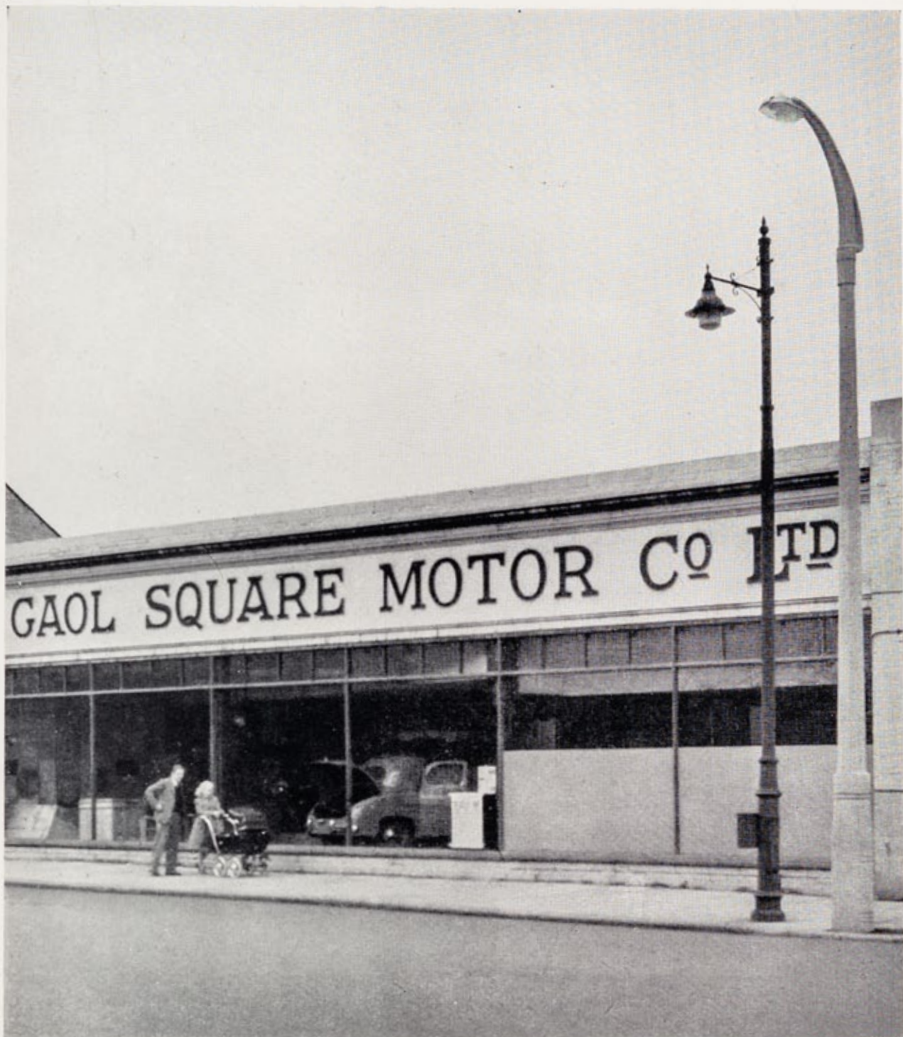
An austere "functional" modern building, with clear and forceful lettering. The size of the letters is to be justified by the fact that the building stands in an open space and not in a narrow street.
