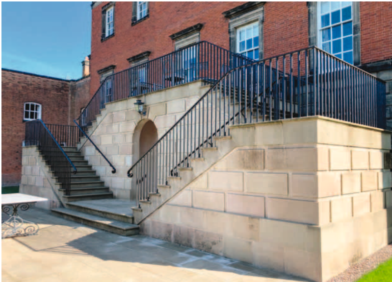
Fig. 19. The new north perron, designed by Peregrine Bryant architecture. ( Peregrine Bryant )
