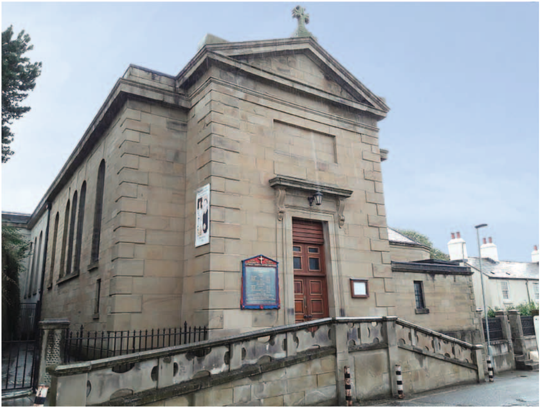
Fig. 5. St. Winefride's Church, Holywell, exterior, the re-orientated liturgical west as now seen from Well Street. (Pjposullivan, Wikimedia Commons)
