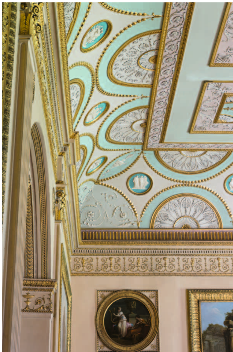
Fig. 2. Detail of the Saloon ceiling at Nostell Priory, with plasterwork undertaken by Joseph Rose & Co. (© National Trust Images/Chris Lacey )
