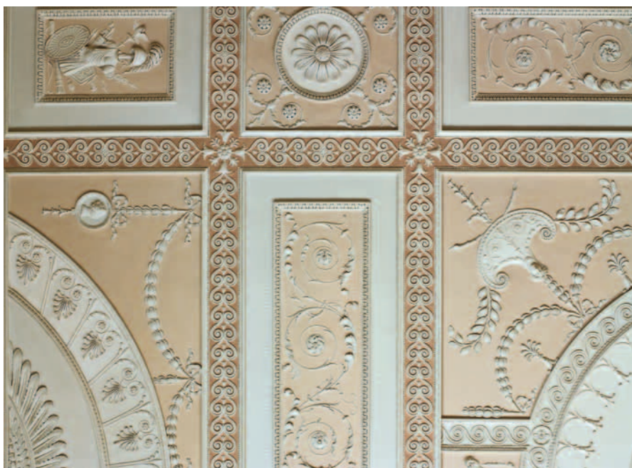
Fig. 4. Detail of Joseph Rose & Co.'s plaster ceiling in the Top Hall. (© National Trust Images/Paul Barker )
