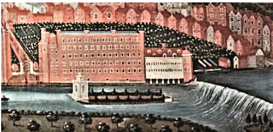
Fig. 3. The Little Byflatt, from Derby Museums' anonymous oil painting of the east prospect of Derby, with the hexagonal angle of Mill House to the right at the end of the weir. ( Derby Museums Trust )
