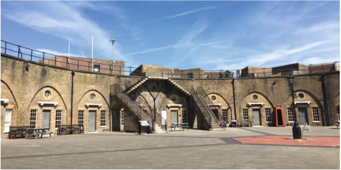
Fig. 13. The Redoubt at Eastbourne, now open to the public, which provided soldiers and supplies to the nearby towers, especially those along Pevensey Bay. ( Author's collection )
