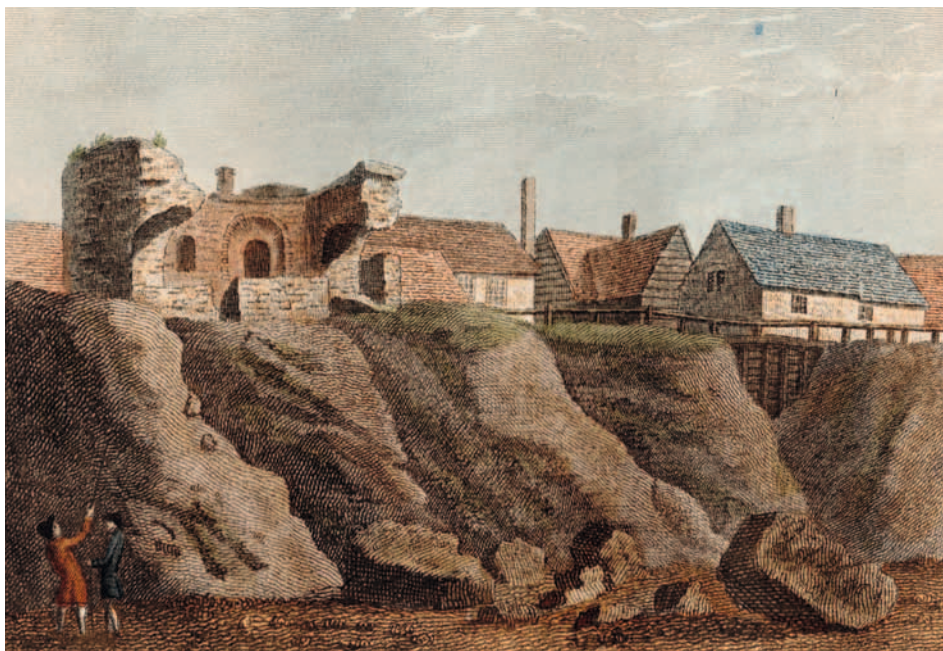
Fig. 6. Erosion at Brighton; the Battery, built in 1759 but useless by 1773, the date of this engraving. ( Author's collection )
