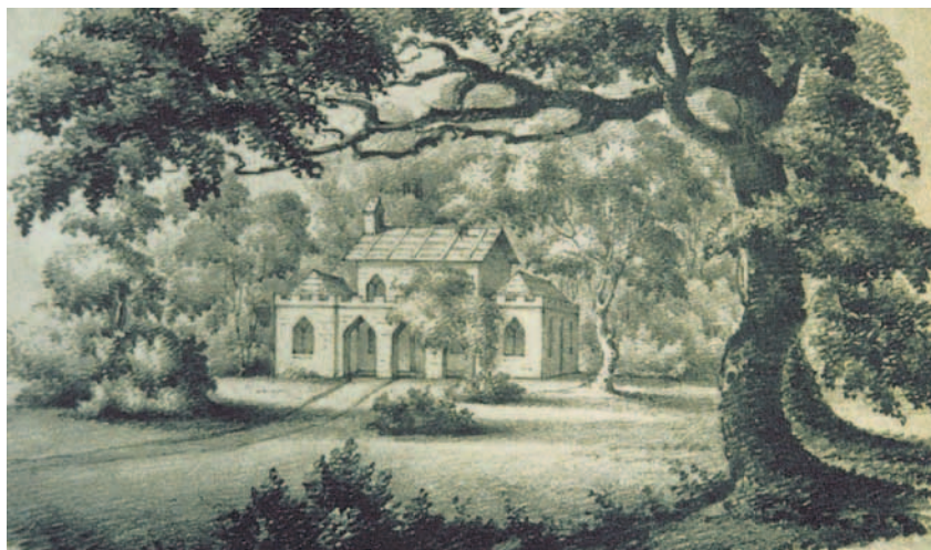
Fig. 13. Sketch of the Dairy from the north-west, c.1830. The patented roofing is clearly shown, although the drawing is inaccurate in form of the side roofs. (Private collection)
