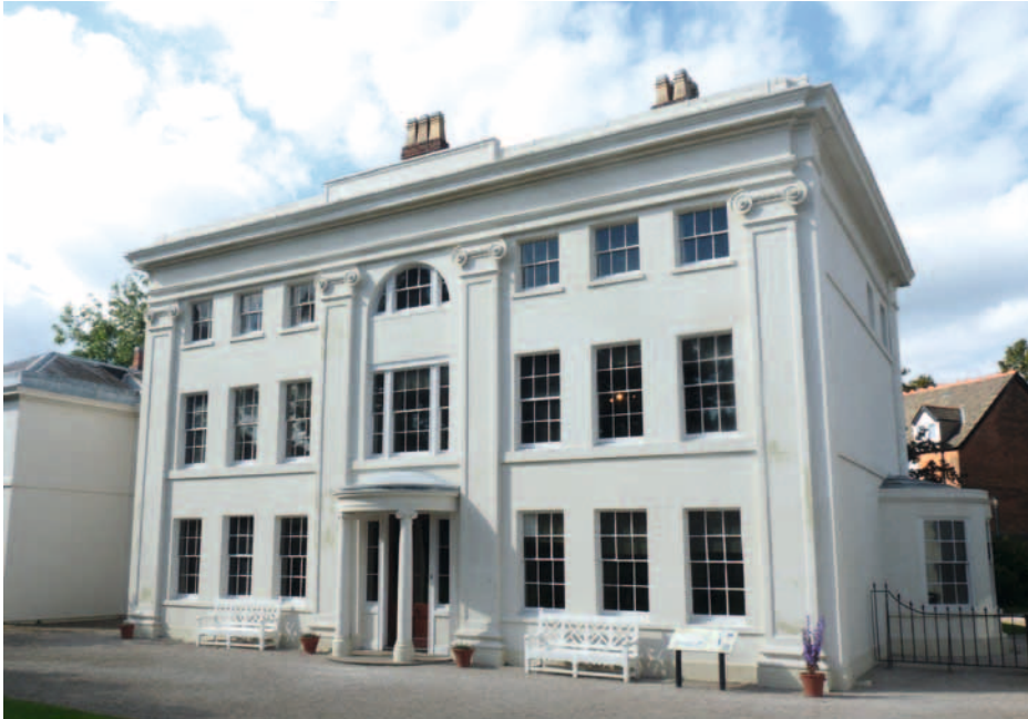
Fig. 16. Soho House, Harmondsworth in Birmingham. This principal elevation is entirely faced in slate, finished in sanded paint. ( Author )
