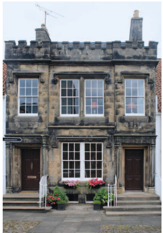
Fig. 3. Main façade of Maspie House, Falkland, Fife. Early nineteenth century. (Photograph: Peter N. Lindfield)
