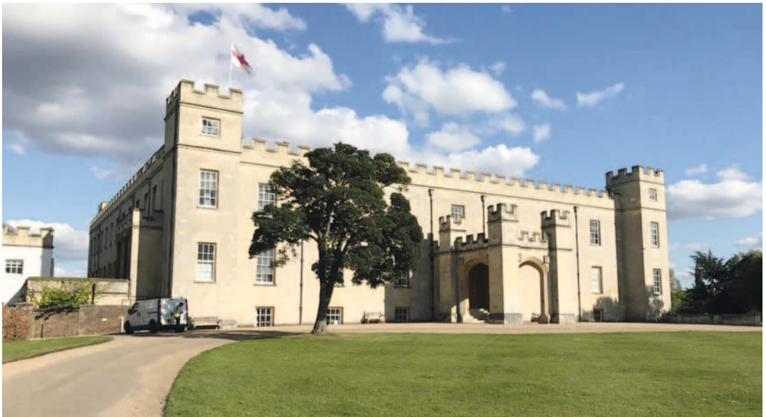
Fig. 1. The exterior of Syon House, as it exists today. ( Author, April 2017 )
