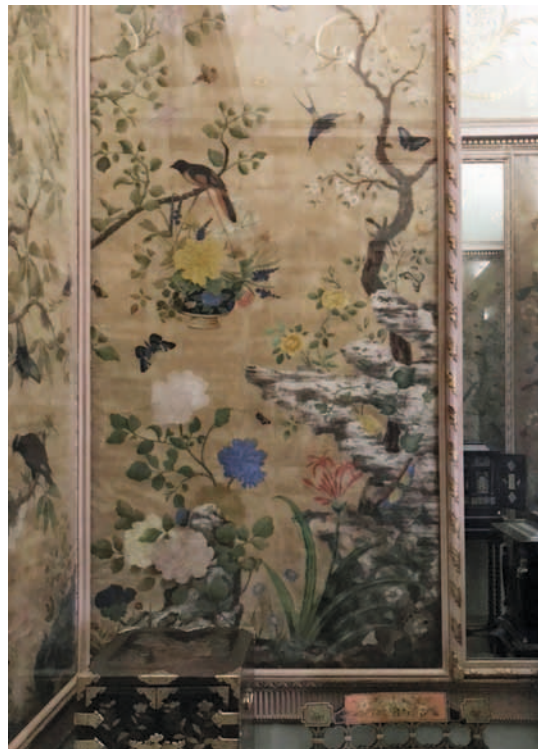
Fig. 13. To the right of a silk panel one of two unadorned looking-glass panels in the south-east Closet, as it exists today. (Author, March 2020)
