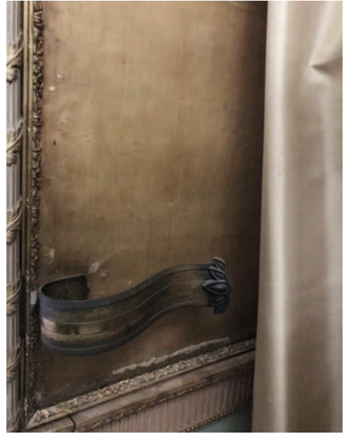
Fig. 15. Detail of the wall behind the curtains depicting tie-back hardware on what is thought to be the lining of the original silk wall panels. (Author, March 2020)
