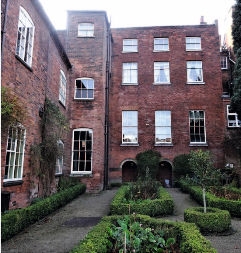
Fig. 17. The restored portion of the garden, looking towards the rear elevation. Note the loggia, centre, post 1850 water closet tower, left of centre, and the 1812-13 rebuilt kitchen, left, 2016. (Derby Museums Trust)
