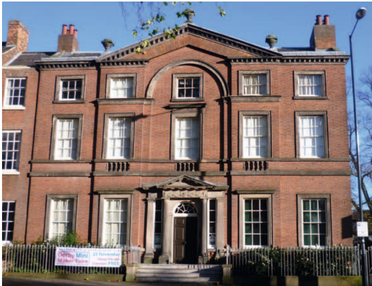
Fig. 1. Pickford's House, street front, 19 November 2013. (M. Craven)
