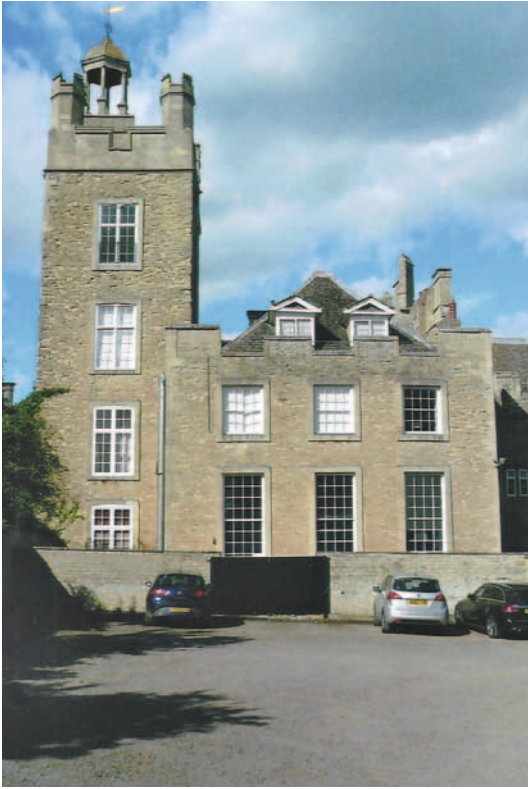
Fig. 7. The ‘new’ 1702 tower and the kitchen with its pyramidal roof. ( Author )
