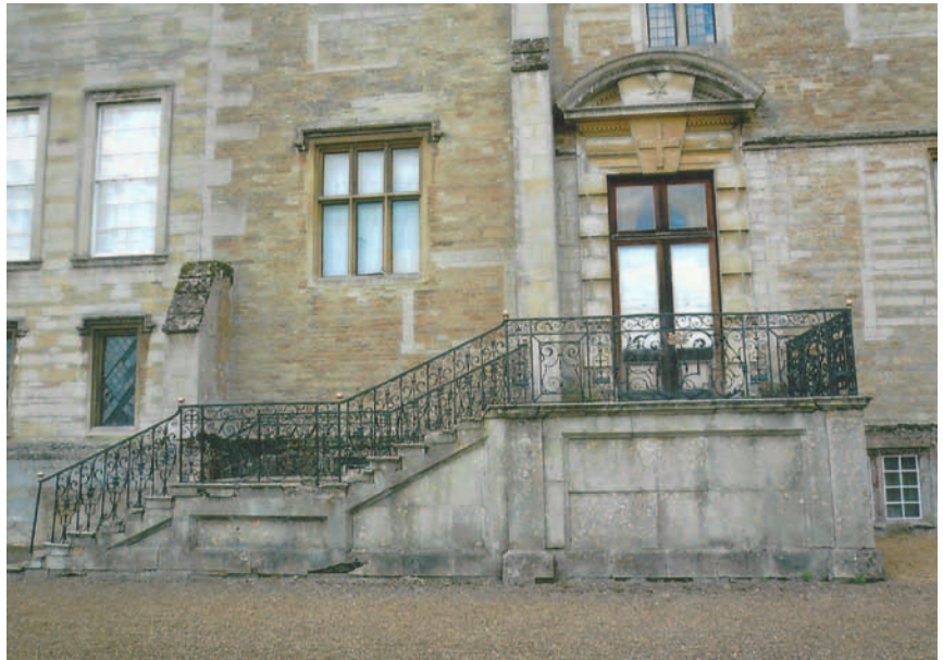
Fig. 8. The north front with the Talman doorcase and garden steps, also showing to its left the base of the 1580s staircase tower and evidence of the pre-1700 window arrangement. ( Author )
