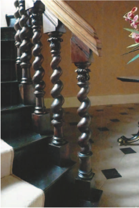
Fig. 13. Drayton House, the final baluster of the Walnut Stair. (Author)
