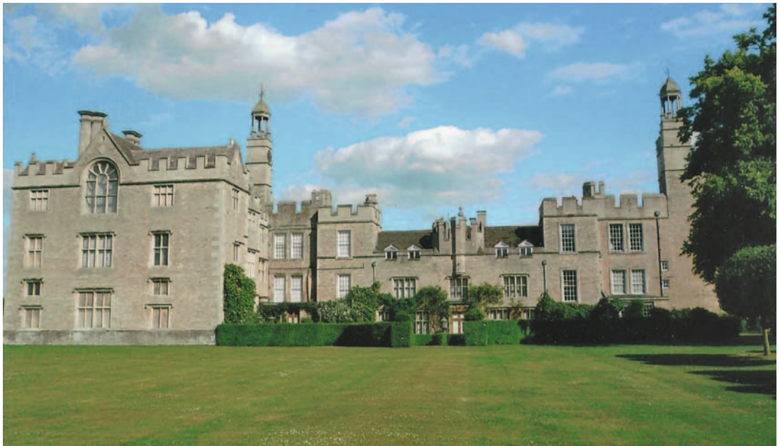
Fig. 1. Drayton House, the complete west front. From left to right: The 1580s wing and tower behind; the two bay medieval solar/undercroft; the Stone Staircase tower; 1580s infill; centre the battlements of the medieval porch; 1580s infill; Oak Staircase tower; two bays c.1700; far right the new c.1700 tower. ( Author )
