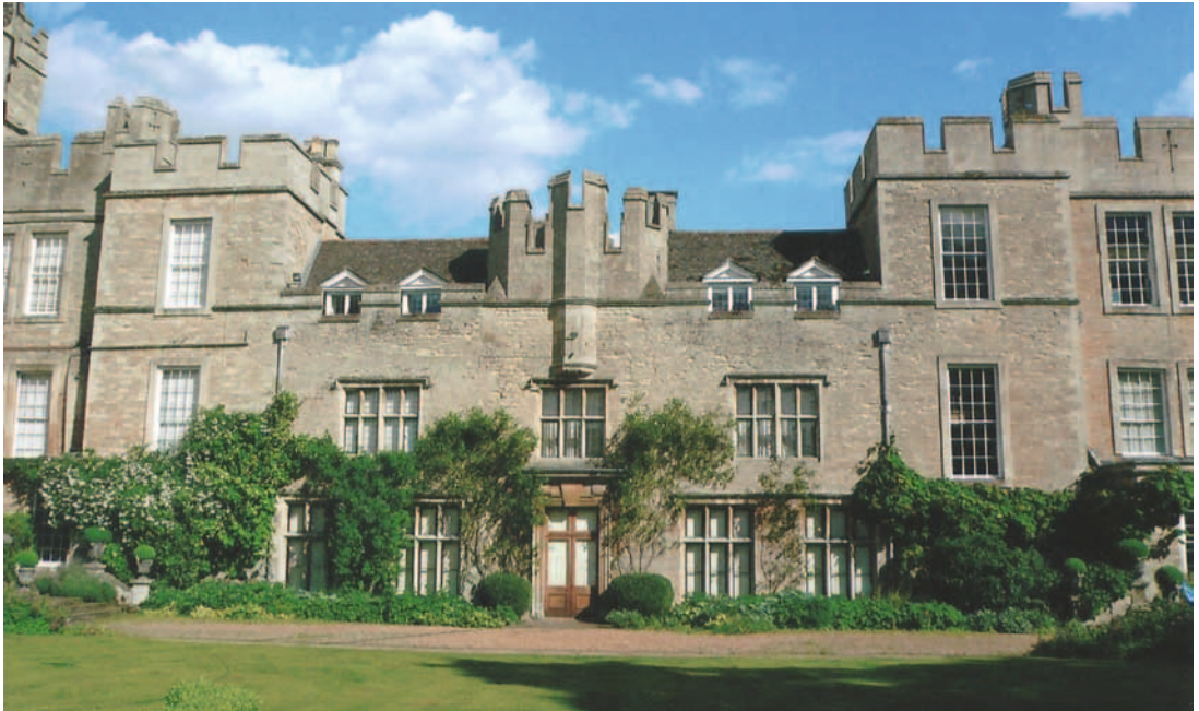
Fig. 3. The centre of the west front. The former medieval porch is at the centre, with Talman's doorcase and the two staircase towers left and right. The ground floor windows were rectangular sash windows of c.1700 until their replacement in around 1900. (Author)
