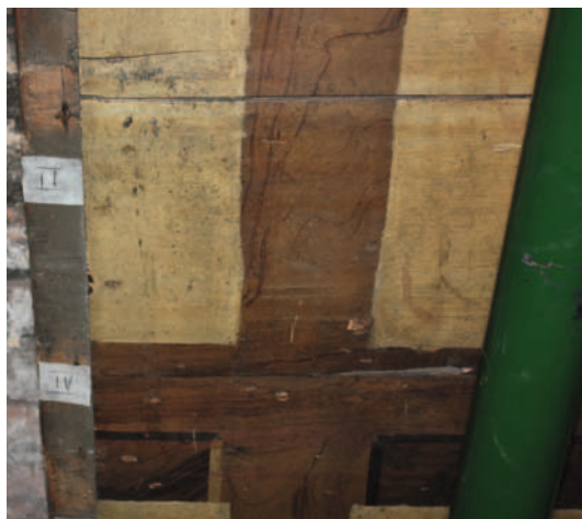
Fig. 8. Tower Green No. 5, walnut-grained panelling, detail of joints. ( Historic Royal Palaces )
