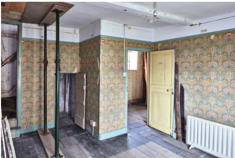
Fig. 2. Tower Green No. 5, closet adjoining the south room, 2nd floor. ( Historic Royal Palaces )
