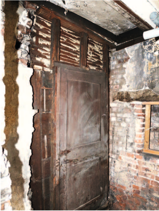
Fig. 5. Tower Green No. 5, late 17th-century door in the north room, ground floor. ( Historic Royal Palaces )
