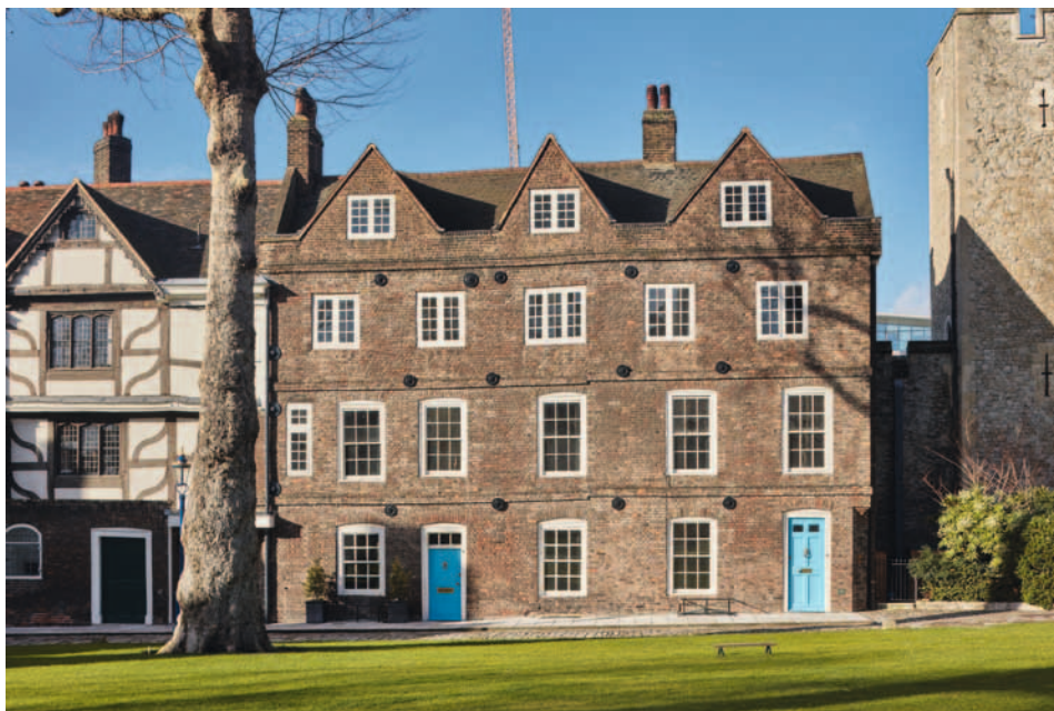
Fig. 1. Houses at Tower Green Nos. 4 & 5, exterior view. ( Historic Royal Palaces )
