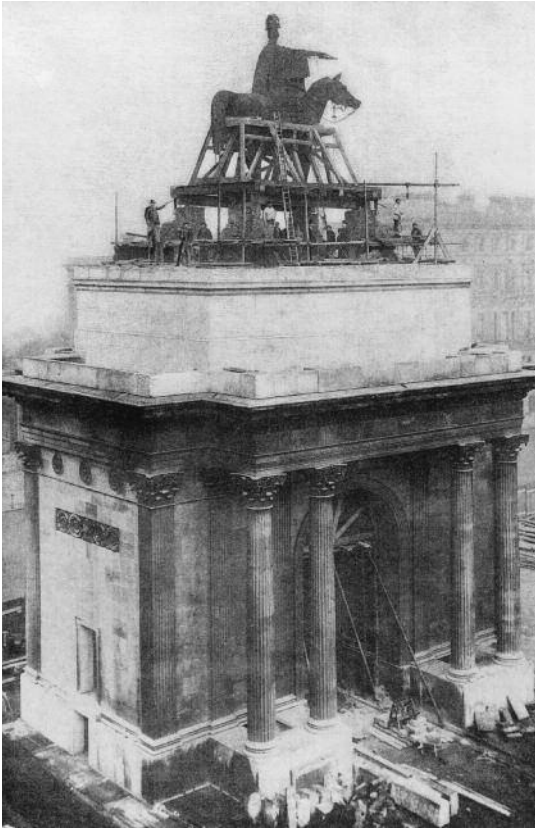
Fig. 37. The Wellington Arch, with the statue about to be lowered, photograph in The Builder , 1883. English Heritage .
