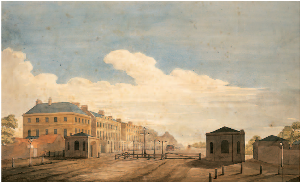
Fig. 17. George Underwood, view of the turnpike gates and lodges at Hyde Park Corner, designed by John Groves junior for the Kensington Turnpike Trust: made for John Soane's Royal Academy lectures, c.1809. The Trustees of Sir John Soane's Museum.
