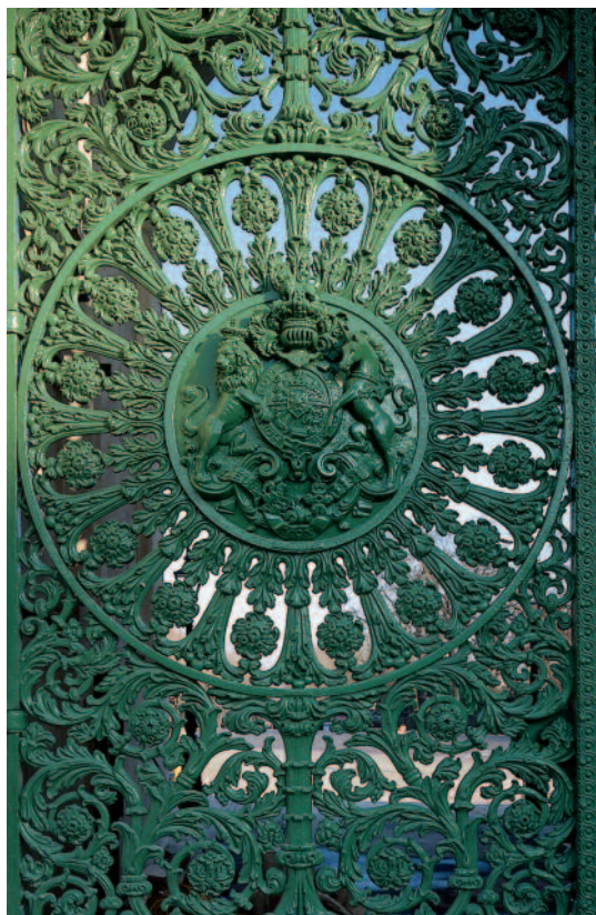
Fig. 33. Wellington Arch, view of the gates made by Bramah and Sons, 1828-9. English Heritage.
