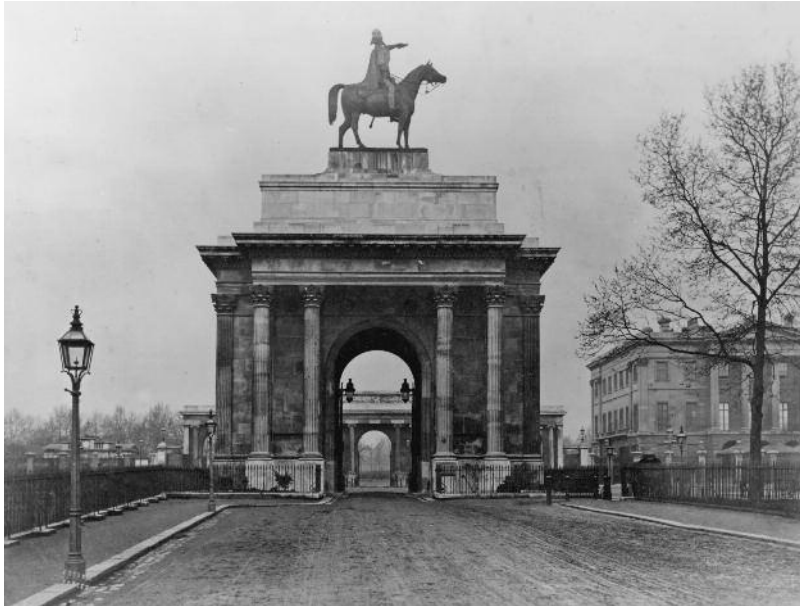
Fig. 35. Photograph of the Wellington Arch with the equestrian statue of the Duke of Wellington, undated, c.1850–60'. English Heritage .
