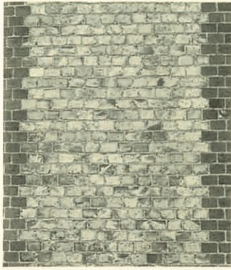
SPOT THE DIFFERENCE: ABOVE - WELL-LAID, THINLY-JOINTED VITRIFIED HEADERS WITH RED BRICK DRESSINGS; BELOW - GEORGIAN BRICKWORK RECENTLY REPOINTED, LEAVING OVERSIZED, UNSIGHTLY MORTAR JOINTS
