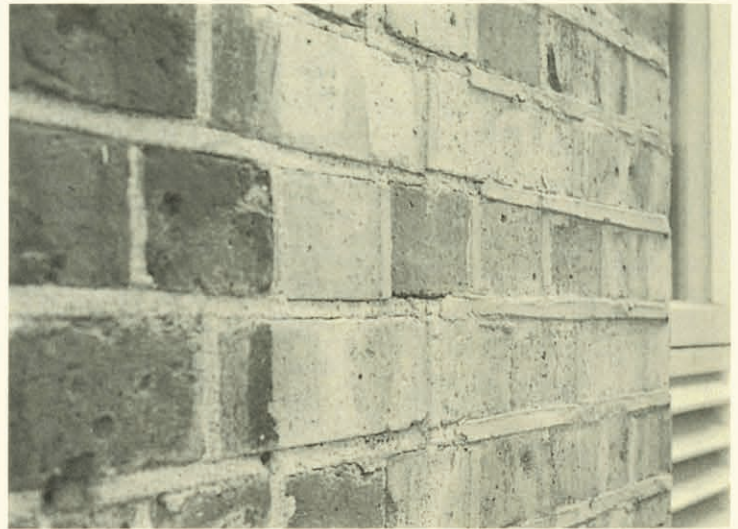
EXAMPLES OF APPALLING MODERN POINTING: LEFT, UNSIGHTLY REPOINTING OF THE LOWER HALF OF A GEORGIAN WALL (LAID IN ENGLISH GARDEN WALL BOND); RIGHT, RIBBON POINTING, PROVIDING RIDGES WHERE WATER CAN COLLECT AND SUBSEQUENTLY PENETRATE INTO THE VULNERABLE BRICK.
