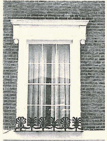
TYPICAL SIX-OVER-SIX PANE SASH. COMPARE WITH THE UPVC REPLACEMENTS BELOW AND OVERLEAF.
