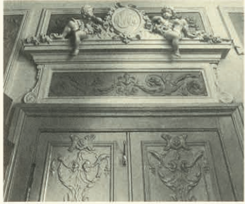
DETAIL FROM A CARTON PIERRE MANUFACTURER'S SHOWROOM IN NORTH LONDON
