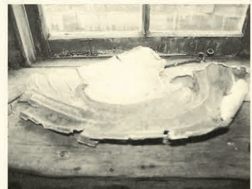
A FRAGMENT OF GILDED PAPIER MACHE FROM GREAT WITLEY. THE BACK REVEALS WHERE IT HAS BEEN PRESSED INTO THE MOULD.
