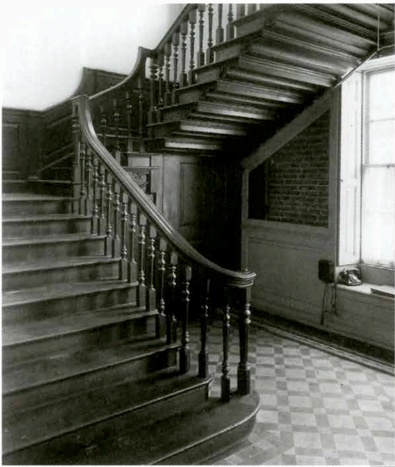
8. LANCASHIRE COURT, LONDON A short run of steeply-raked stairs in a modest town house, with a completely plain newel post, moulded handrail and a closed string with three different balusters, of which the middle one is the original pattern. (photo Georgian Group)
