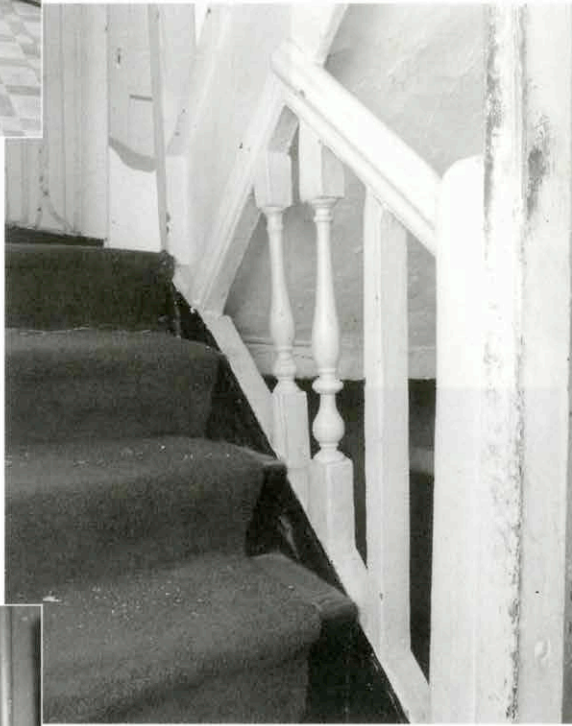
7. WILMER HOUSE, FARNHAM SURREY A hardwood stair with a cut string and ornamental tread- ends which are both inlaid and carved; the underside of the stairs is also moulded. Two balusters to each tread, the balusters having tapering fluted shafts, the handrail moulded and ramped up to the corner newel posts. (photo Surrey CC P3503)
