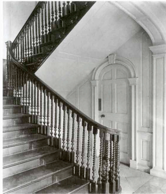
13. WIDCOMBE MANOR HOUSE, BATH A handsome main stair, three twisted balusters to each tread. The handrail is ramped up to the landing and ends with a twist onto the bottom newel. The steps have moulded nosings, typical of the better stairs. (photo NMR DD50/201 Messrs Batsford)
