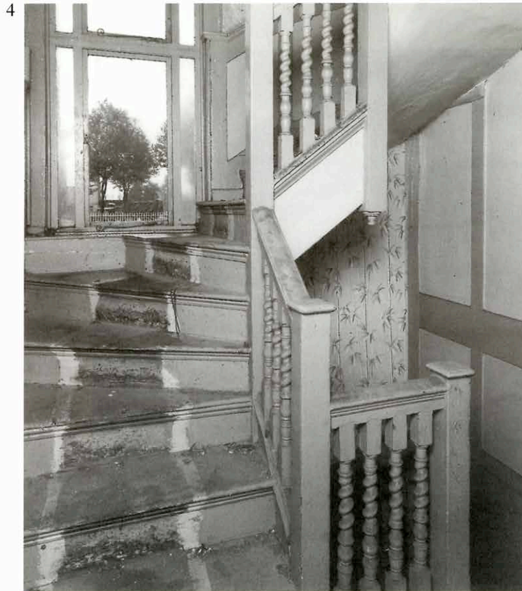
4. ALBURY STREET, DEPTFORD, LONDON A section of a cramped open-well staircase in a modest town house, with winders used to turn the corner rather than a landing. The square wooden newels have simple caps, the handrail has a slightly more elaborate moulding, the twisted balusters are closely- set. ( photo LMA 71/11691 )
