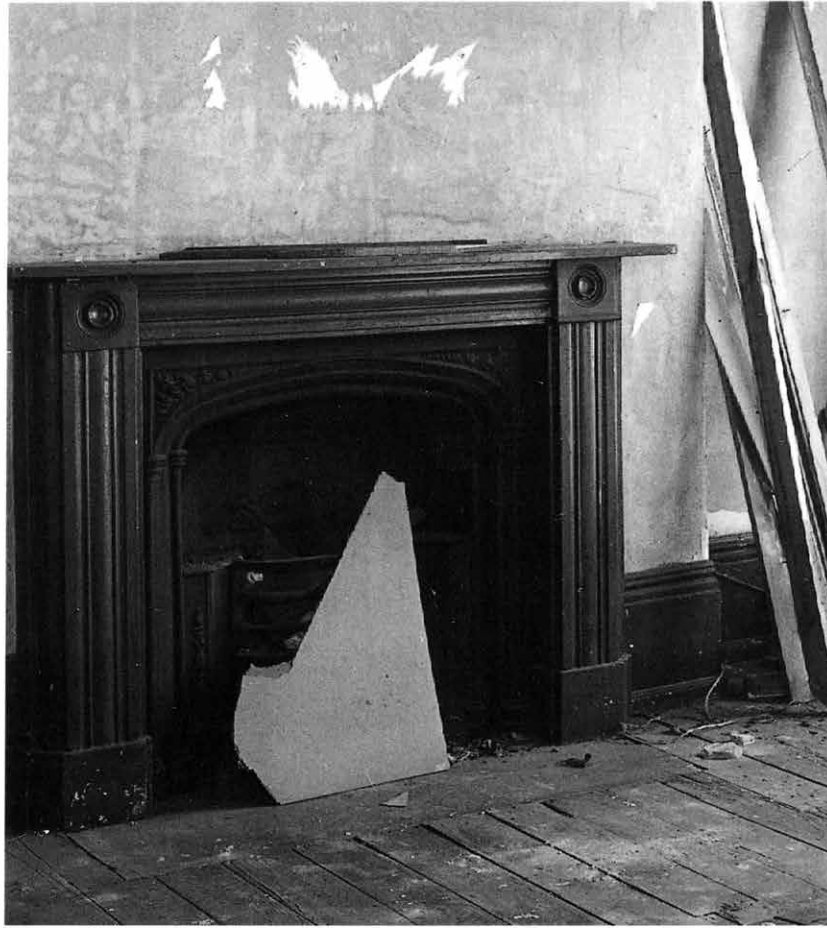
49. LONDON, TREDEGAR SQUARE, L B TOWER HAMLETS: 1st floor front room; a good example of the reeding and roundel type with heavier mouldings than early examples, probably in stone or marble but painted over (photo LMA: ref 73/120/256/6)
