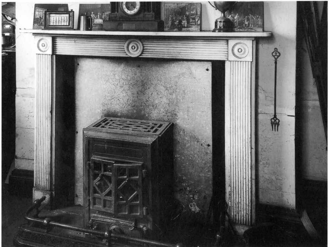
59. NEWTON LONGVILLE, BUCKS: ground floor; reeding and roundel with an additional central roundel ( photo NMR: ref BB63/1175 )
