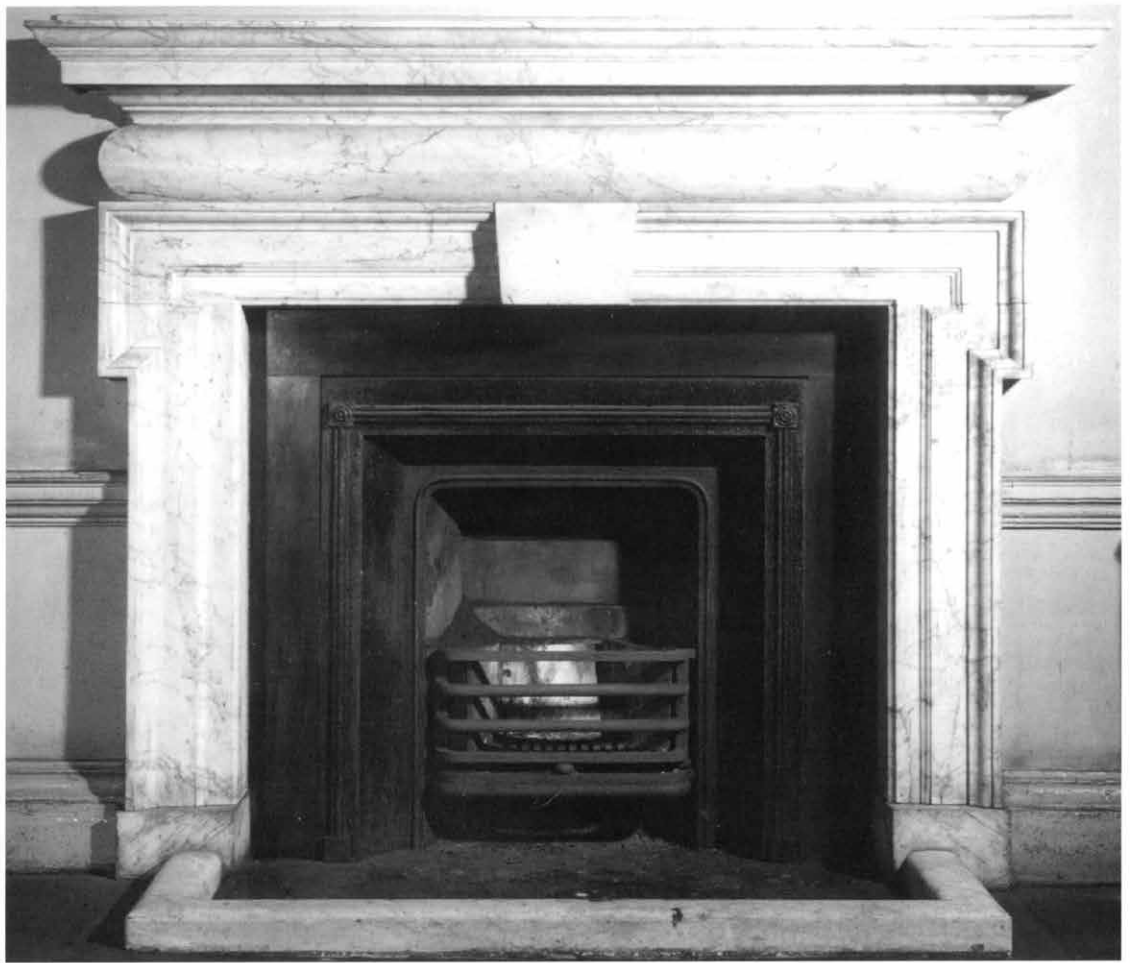
14. LONDON WHITEHALL, Treasury Buildings, designed by William Kent 1737: a handsome eared marble surround with a pulvinated frieze and moulded overmantel (photo NMR: ref W117)
