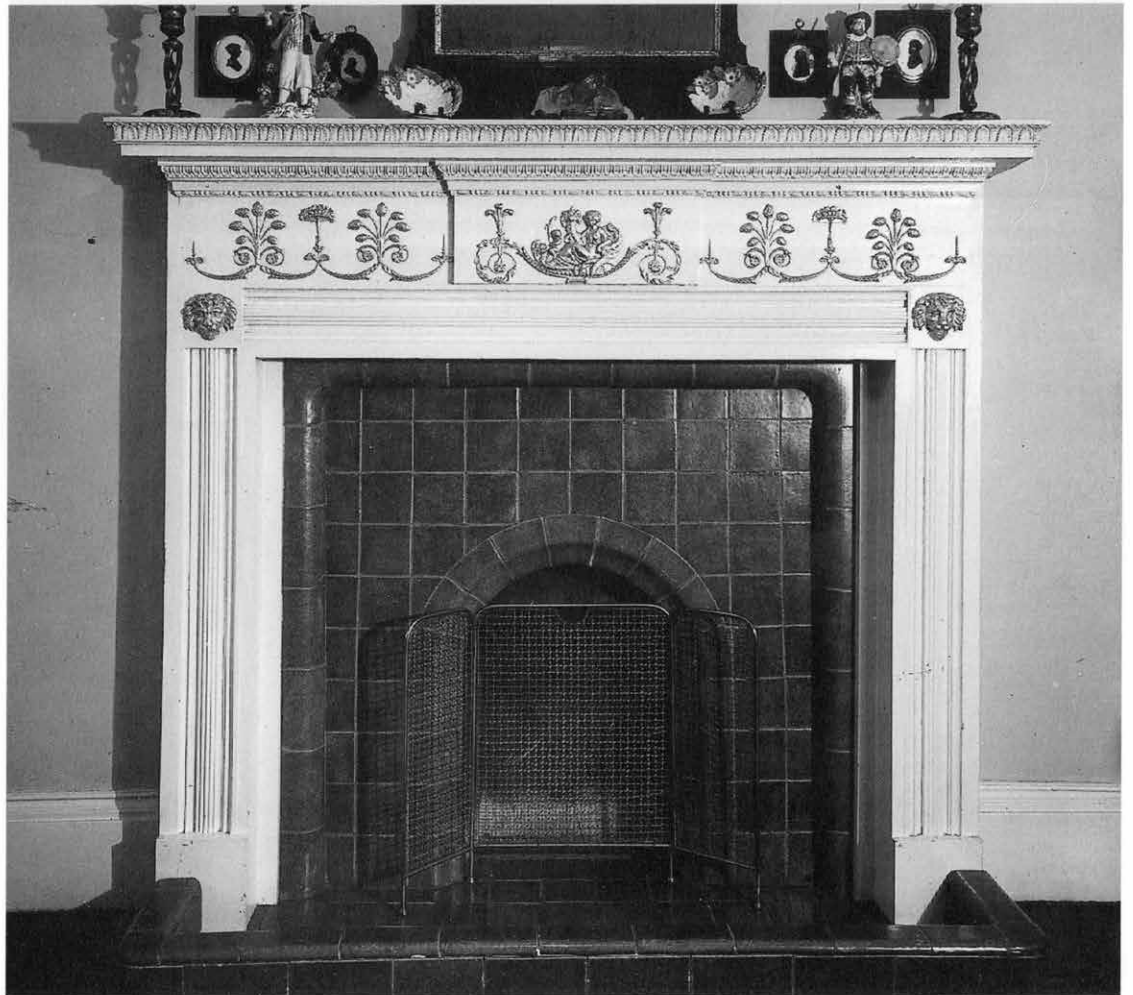
54. BATH, BATHWICK HILL: dining room; a timber chimneypiece with applied composition ornament ( photo NMR: ref AA471/1043 )
